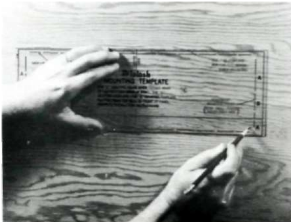
Figure 11. Positioning the Mounting Template Over Proposed Area to be Cutout.
