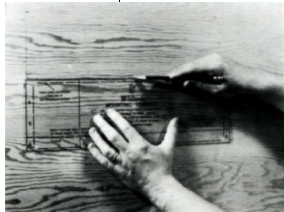
Figure 12. Marking the Cutout Indications.
